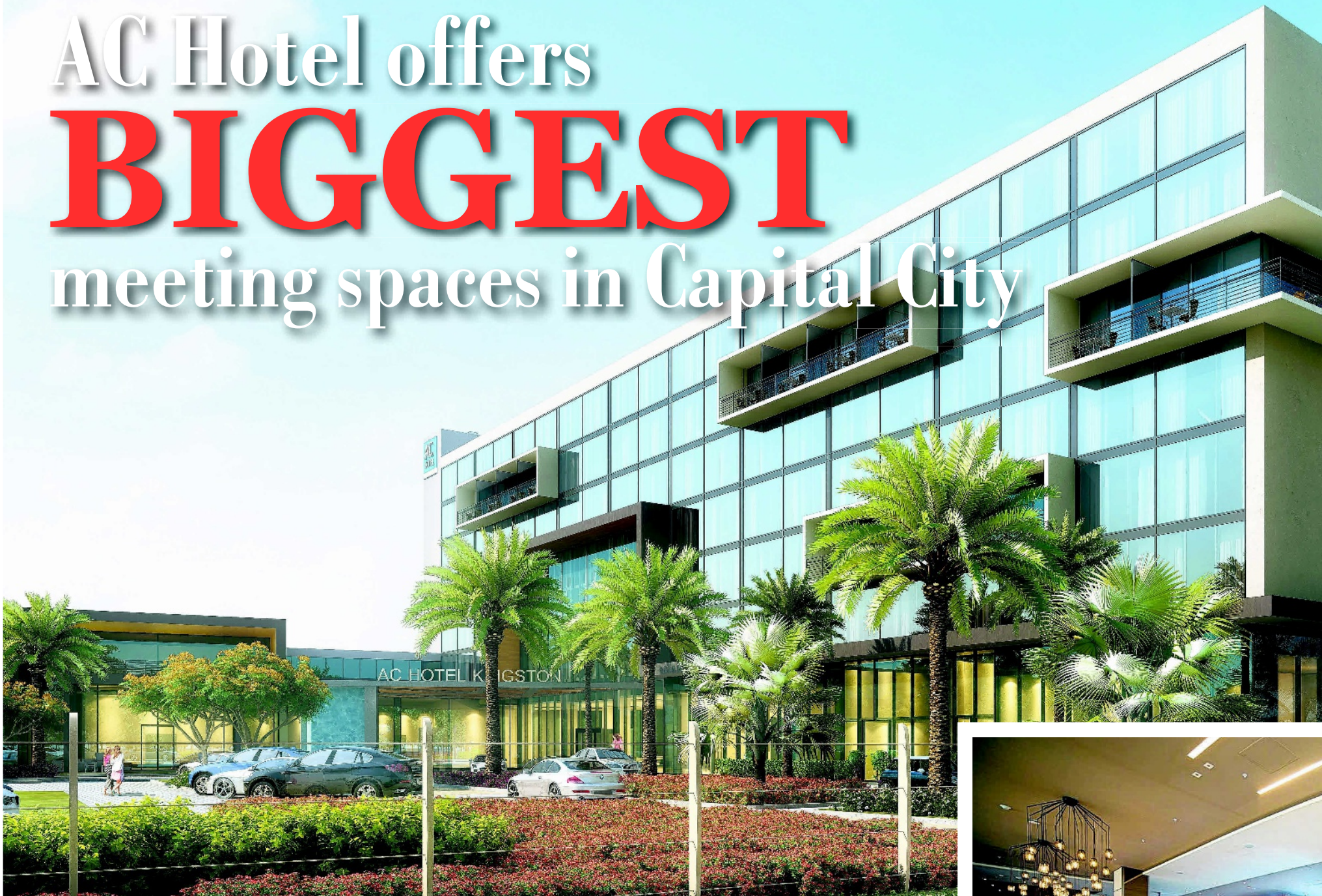
Exterior of AC Hotel Kingston CONTRIBUTED
