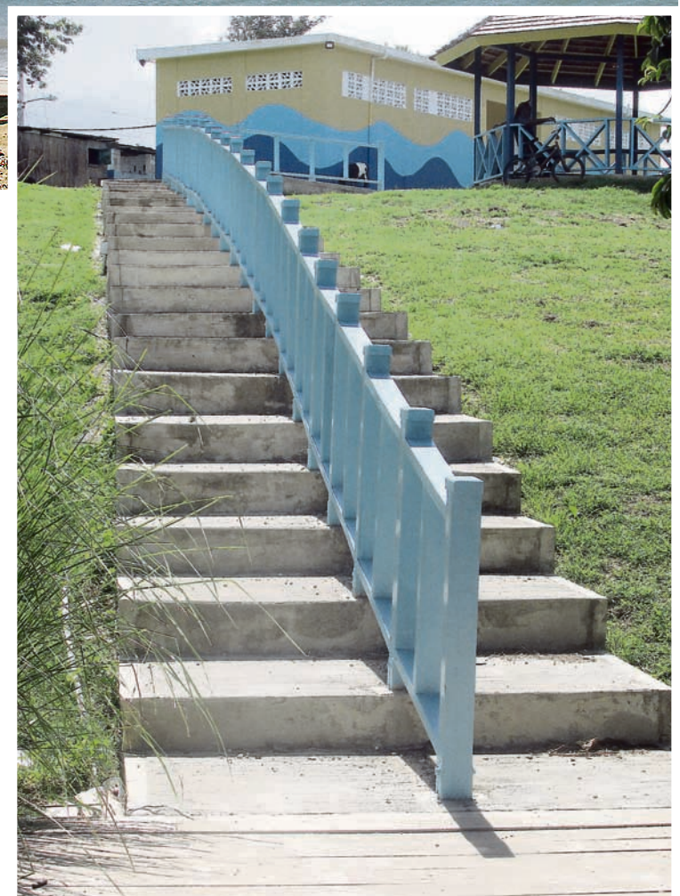
A rehabilitated walkway at the recently upgraded Lyssons Beach.
