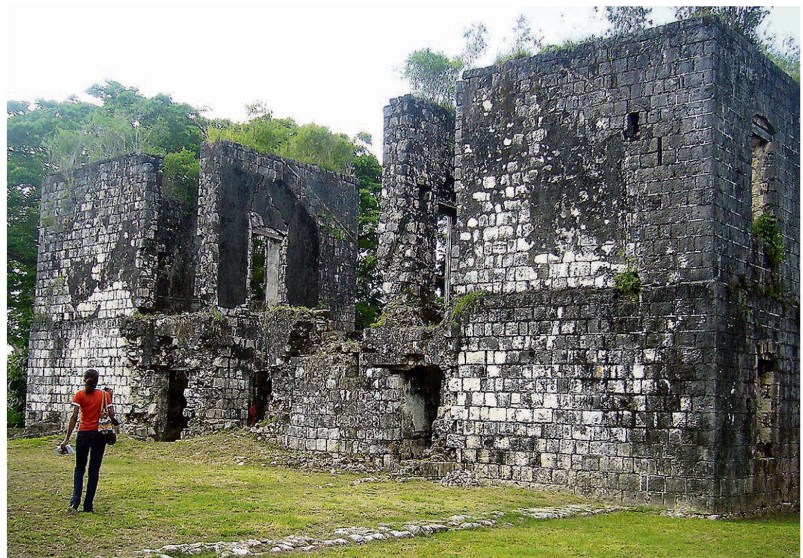
The ruins of the Stokes Hall Great House in St Thomas.
