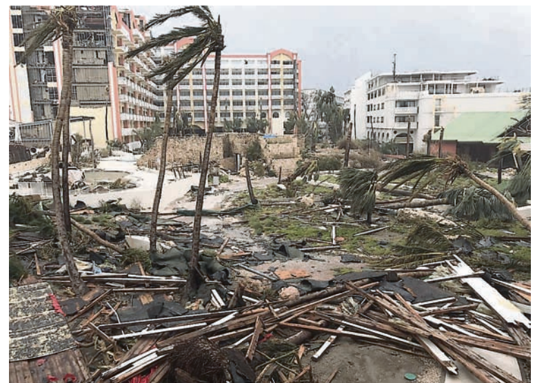
Some of the damage left in St Maarten after it was ravaged by Hurricane Irma.
