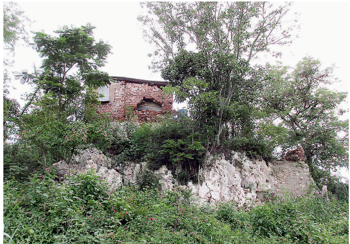
A section of the remnants of Lenard Howell's kitchen at Pinnacle, St Catherine.
