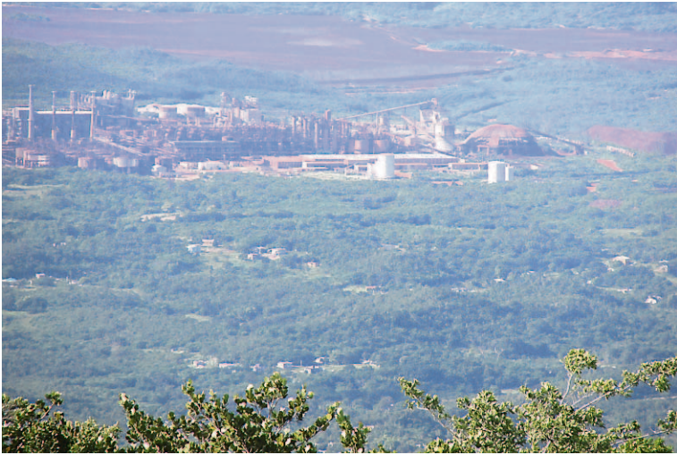
View of an alumina plant in St Elizabeth from Lincoln, Manchester.
