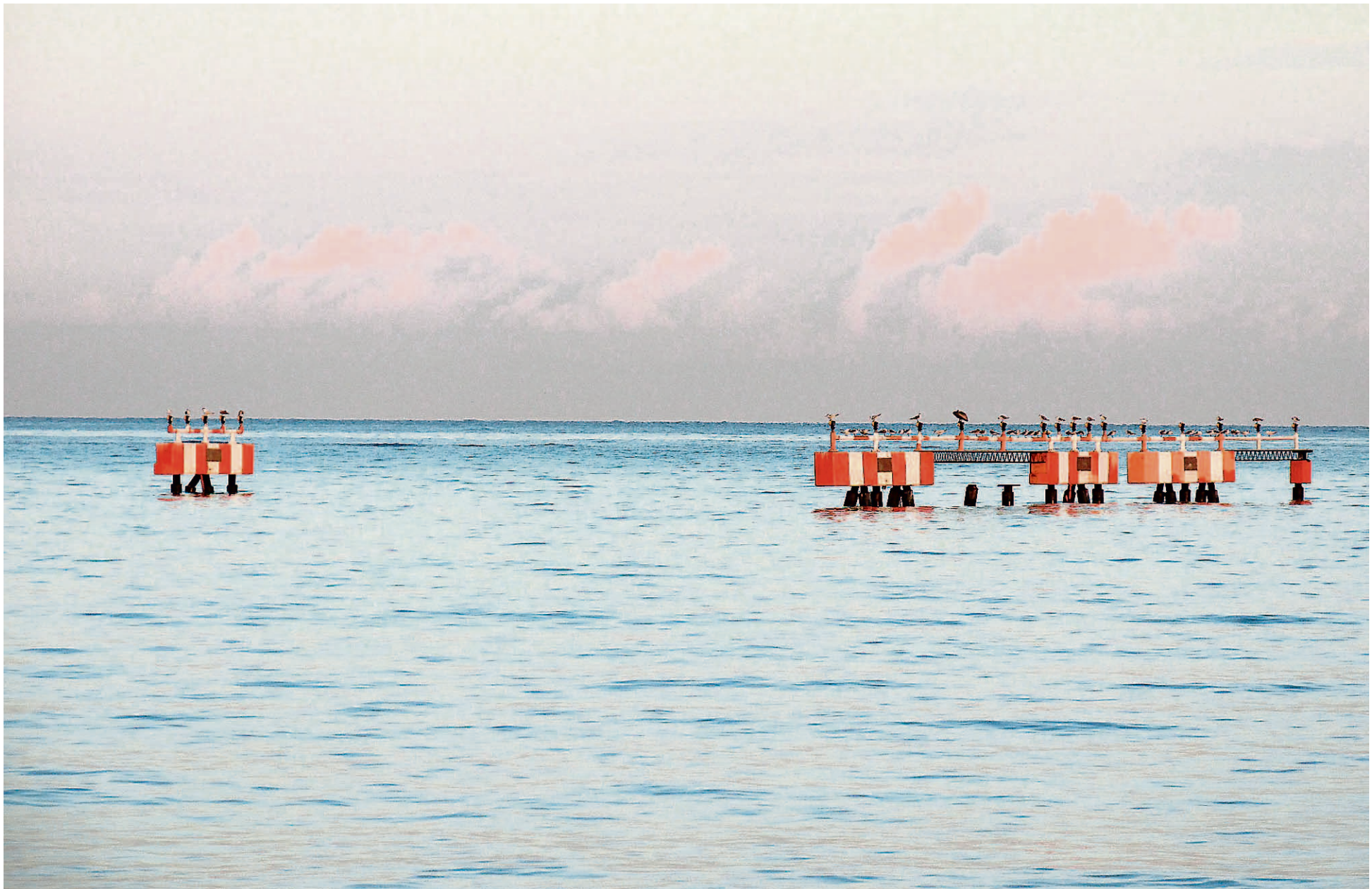
Birds nesting on the lights, which guide descending airplanes to Sangster International Airport in Montego Bay.
