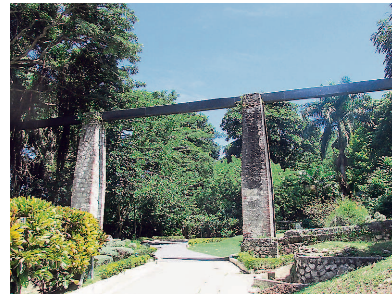
This aqueduct, atop decades-old brick columns, carries water from the Flint River to spin an old waterwheel.
